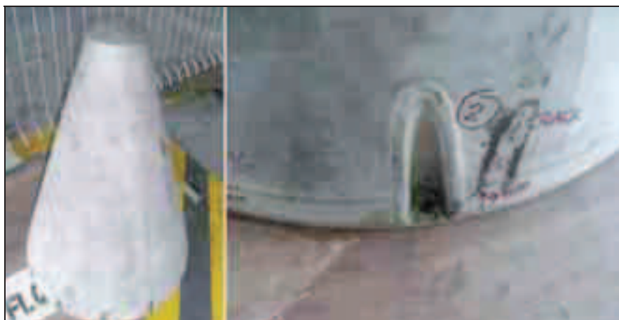
Fig. 1. Crack on the mounting bolt hole of the exhaust cone
