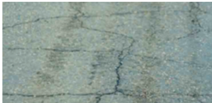
Fig. 9. Alligator cracking [13]
