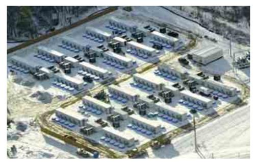
Fig. 8. A 20 MW plant constructed in Stephentown based on flywheels (NY, USA) [8]
