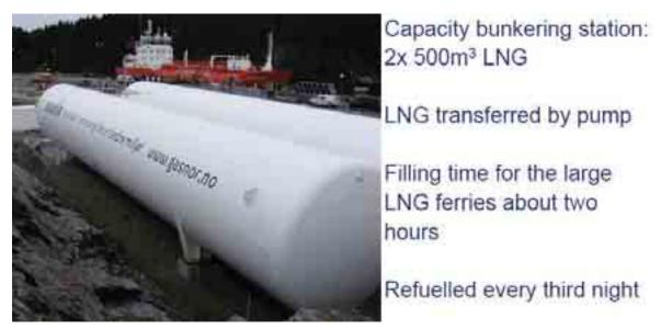
Fig. 5. LNG bunkering station at ferry berth for m/v Bergensfjord [10]
