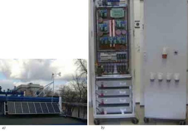
Fig. 2. View of photovoltaic panels (a) and control cubicle (b) of the charging station demonstrator
